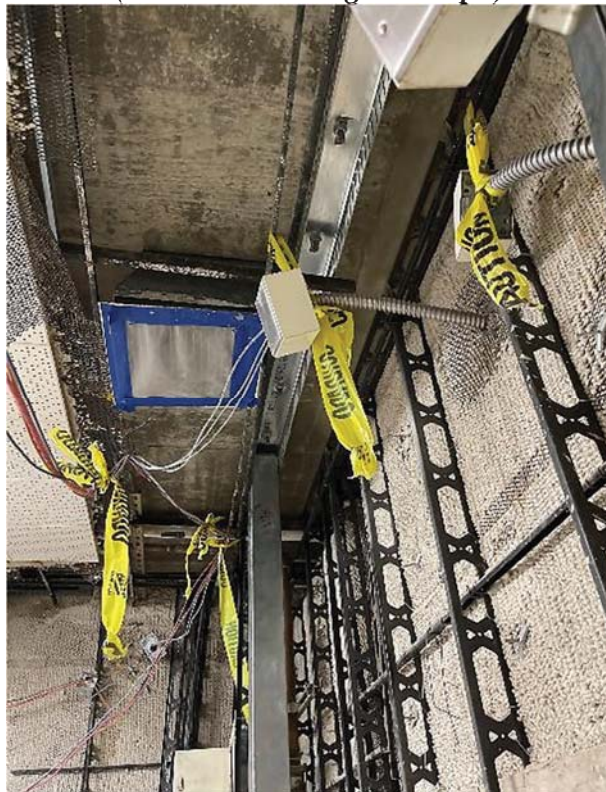
Figure 6. Black Iron Walls at the South Wall of the Girl’s Gym Women’s Restroom (CO T-523 Package Excerpt )
