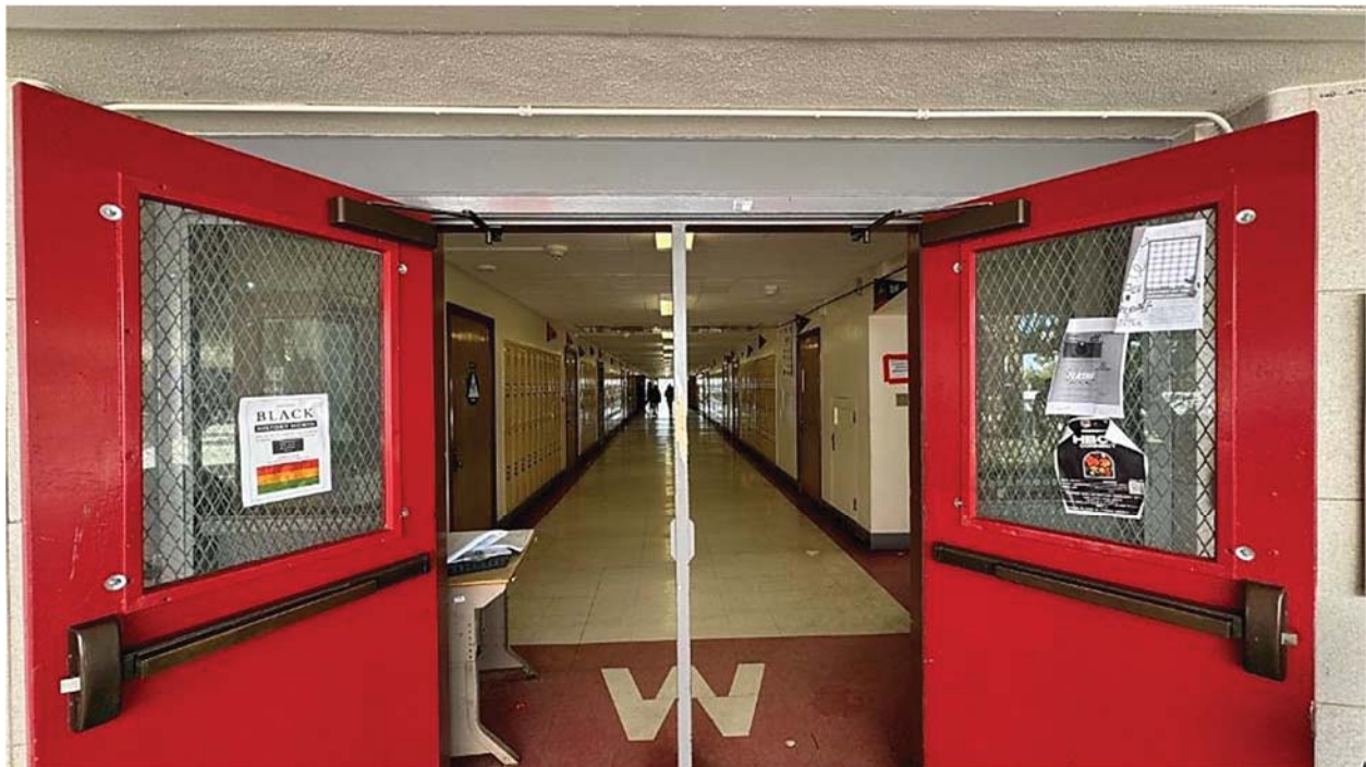
Figure 18. Upgraded Entrance Door Hardware in the Foreign Language Building
