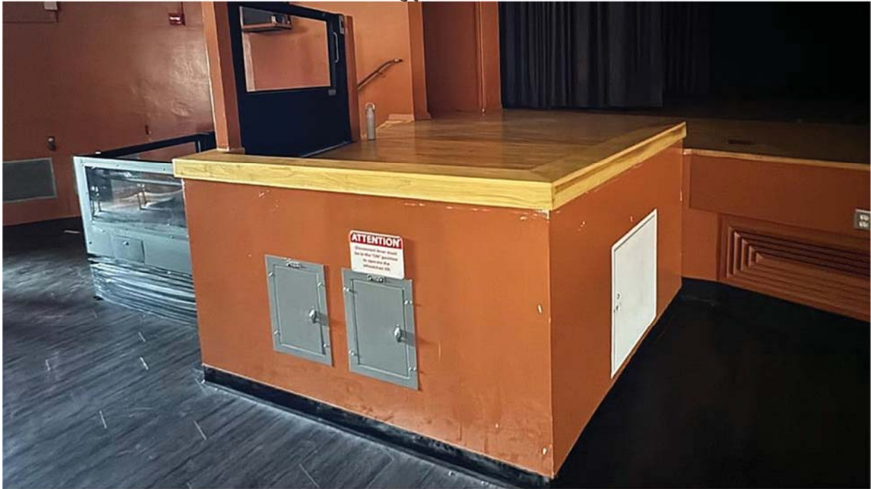
Figure 16. New Maple Cap over Curbs at the Upper Chairlift Landings in the Assembly Building for CO T-567
