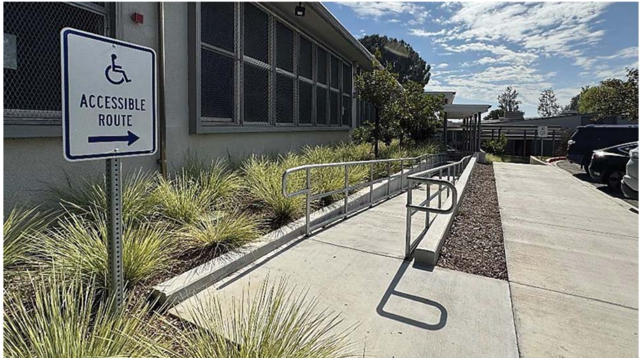
Figure 23. New ADA Concrete Ramp #2 at the Science Building
