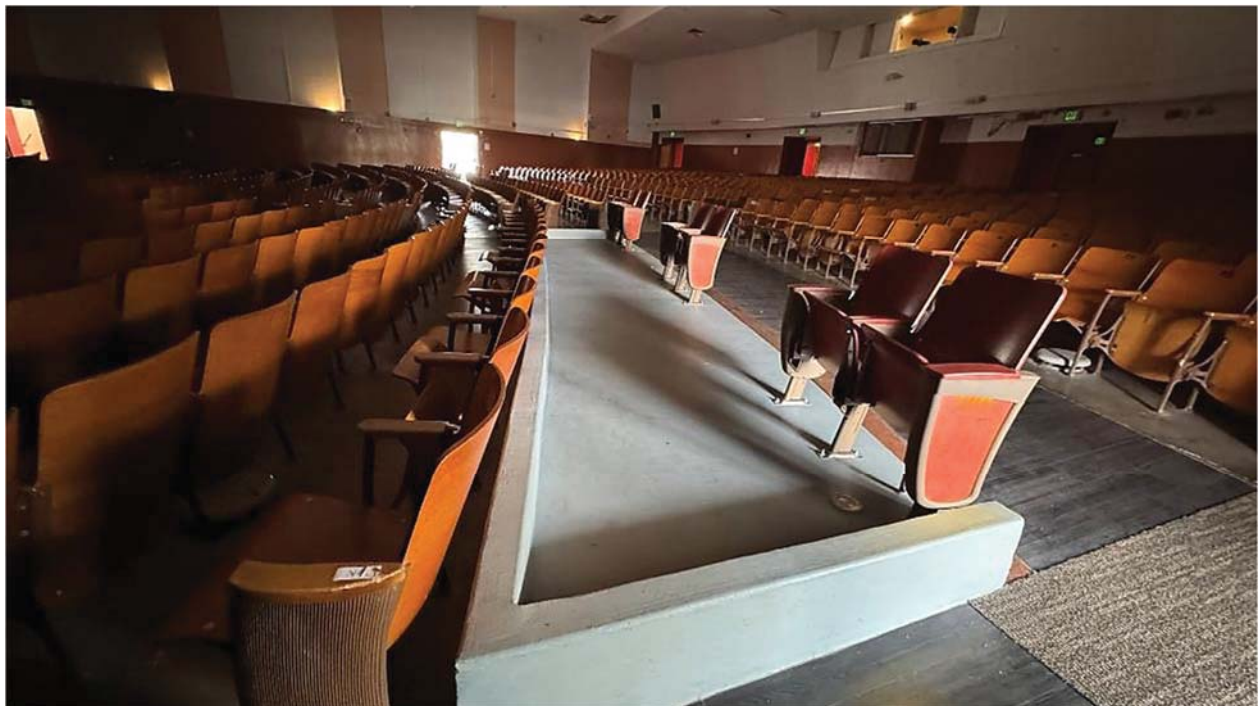
Figure 24. New ADA Seating in the Assembly Building
