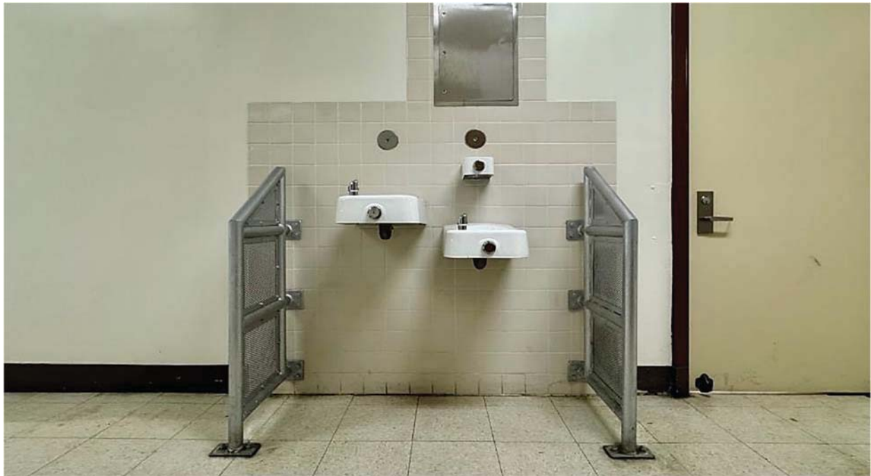
Figure 22. New Accessible Drinking Fountain Installed in the Administration Building
